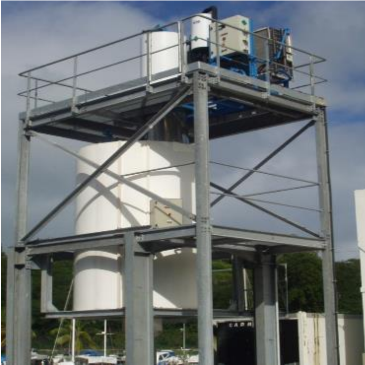
FINAL DESIGN BEFORE CLADDING - Frame and access ladders
